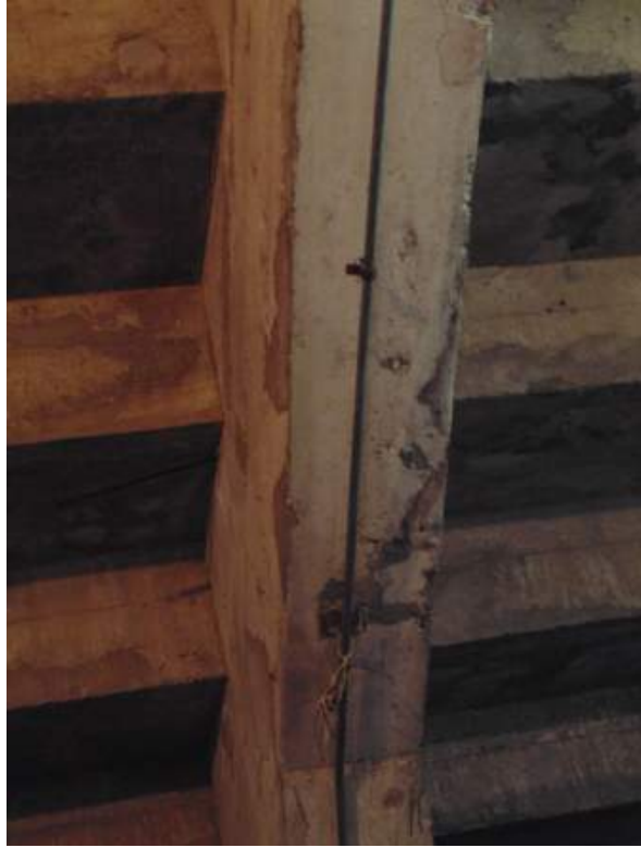
FIGURE C1C: CRACKING/SPALLING IN CONC. GIRDER
