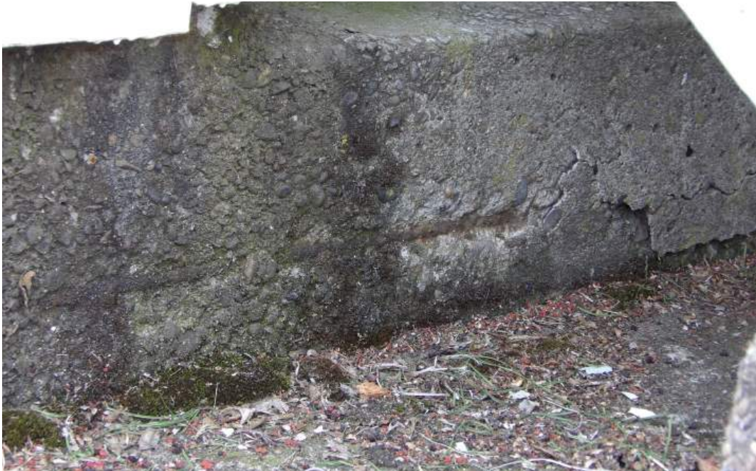
FIGURE F3A: EXPOSED REBAR WITH MINOR CRACKING AND SPALLING
