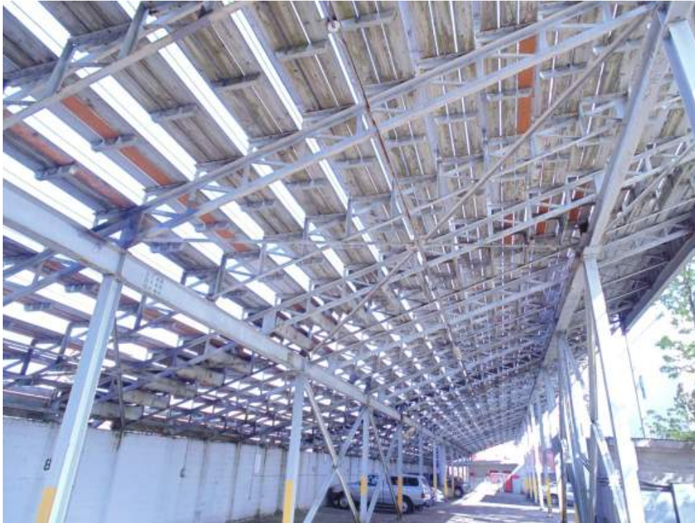
View From Underside of Grandstand
