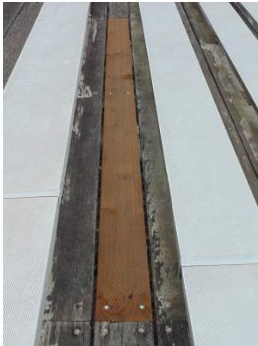
FIGURE B4B: REPLACEMENT PRESSURE TREATED BLEACHER BOARD
