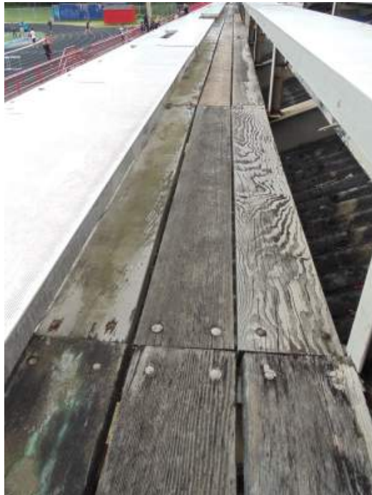
FIGURE B5B: ORIGINAL SINGLE SPAN BLEACHER BOARD
