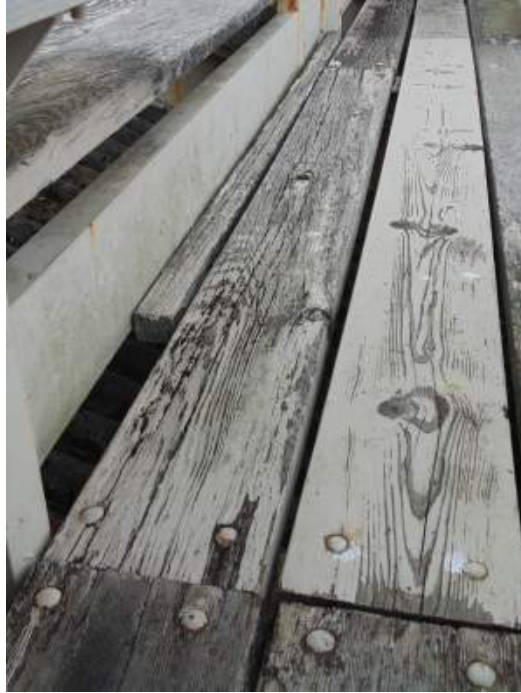
FIGURE B5A: ORIGINAL SINGLE SPAN BLEACHER BOARD
