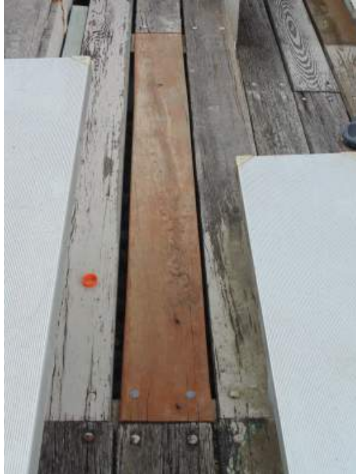
FIGURE B3A: REPLACEMENT CEDAR BLEACHER BOARDS
