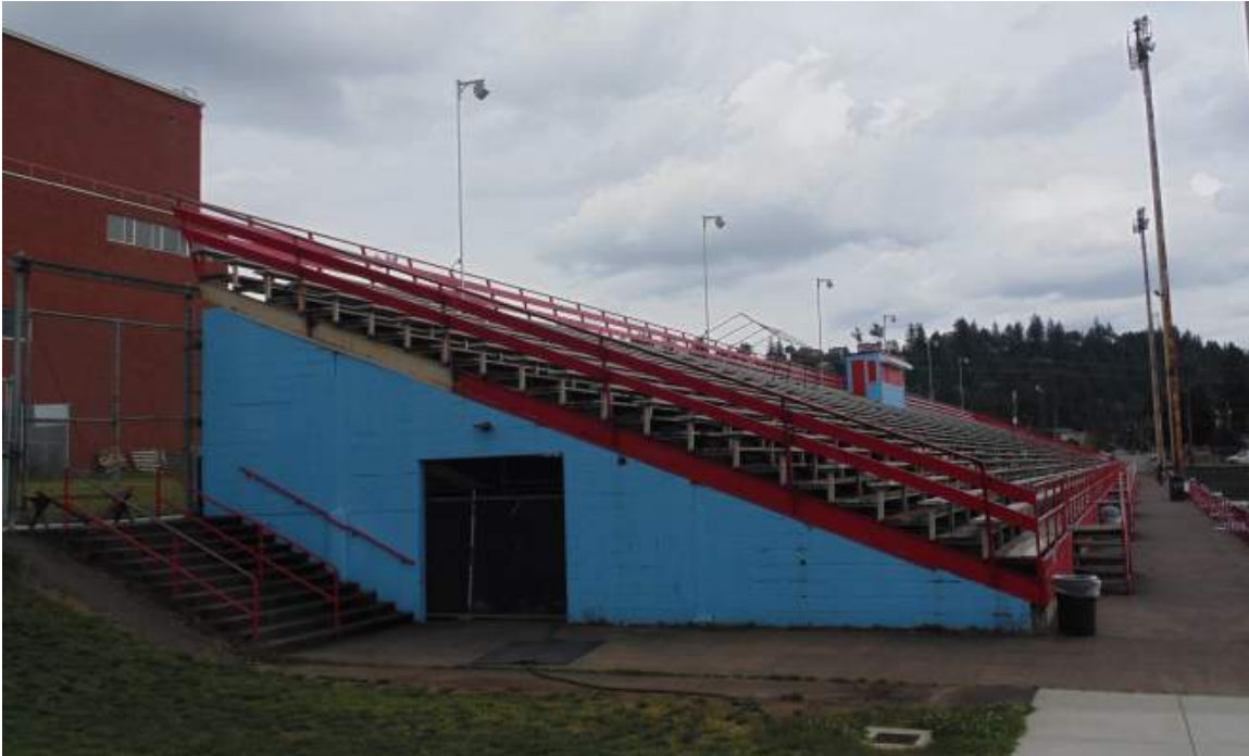
West View of Grandstand
