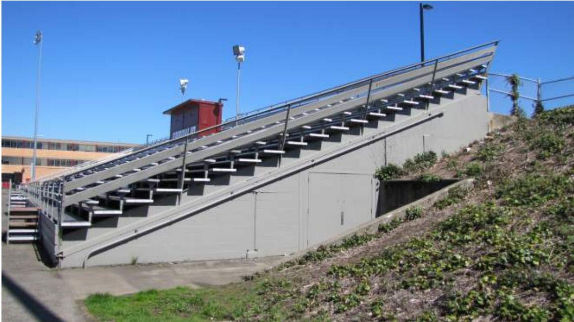
South View of Grandstand
