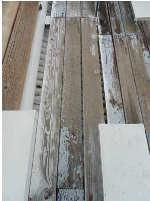
FIGURE B5A: ORIGINAL SINGLE SPAN BLEACHER BOARD
