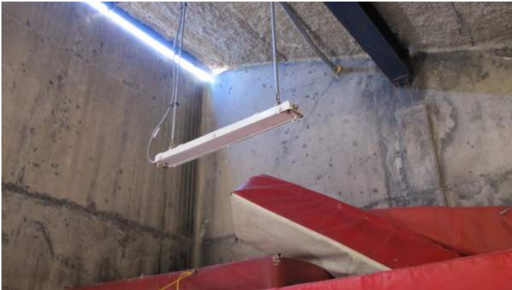
FIGURE F3: SMALL CONCRETE CRACK AT SOUTH WALL PILASTER
