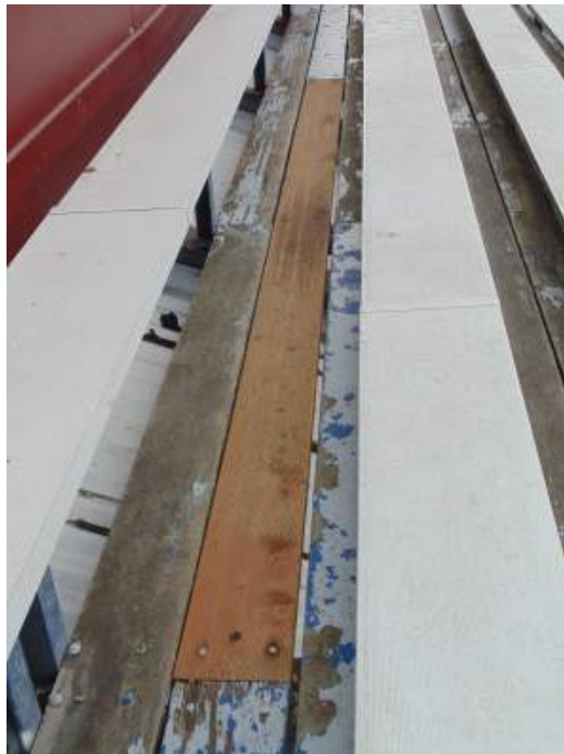
FIGURE B4A: REPLACED PRESSURE TREATED DFL BLEACHER BOARD
