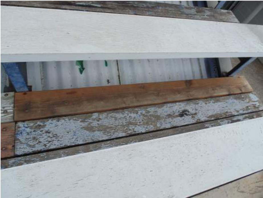
FIGURE B3A: REPLACED CEDAR BLEACHER BOARD
