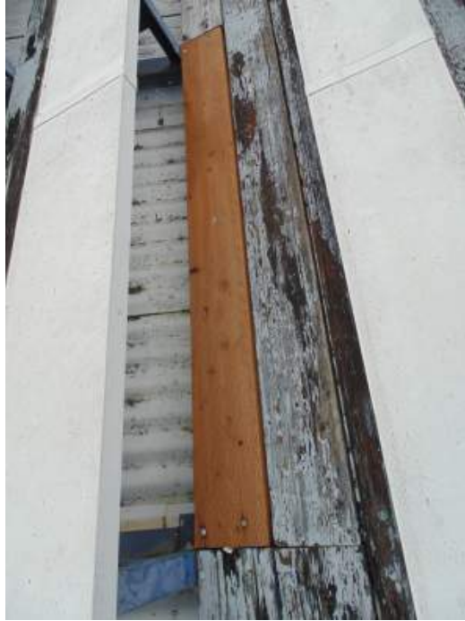
FIGURE B4B: REPLACED PRESSURE TREATED DFL BLEACHER BOARD
