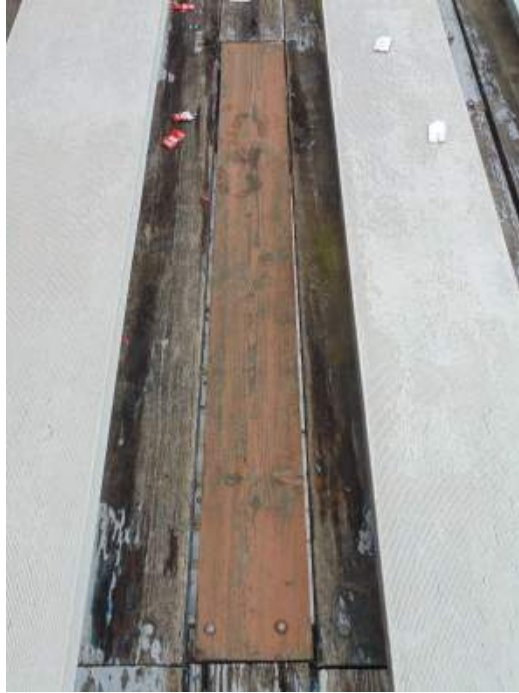
FIGURE B3B: REPLACED CEDAR BLEACHER BOARD
